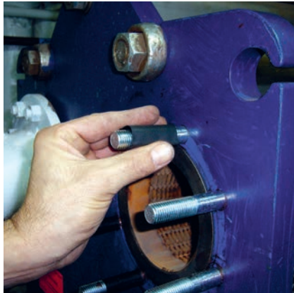
SHUFFLE THE SHRINKING HOSE ABOUT THE BOLT
