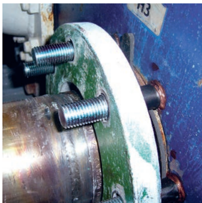
SHUFFLE THE PLASTIC INSULATING DISC ABOUT THE BOLT
